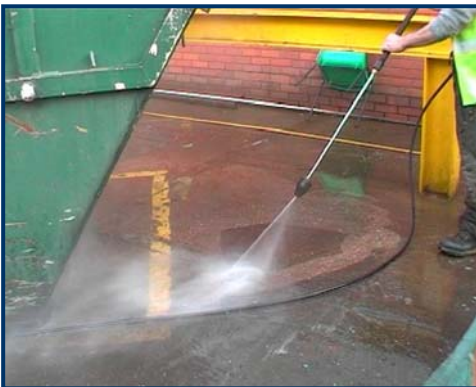
Pressure lance cleaning
