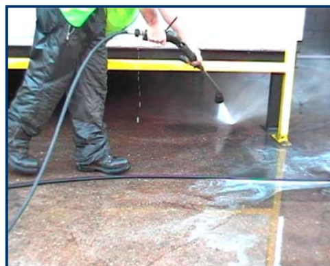
Once clear, the second clean down with pressure lance can commence
