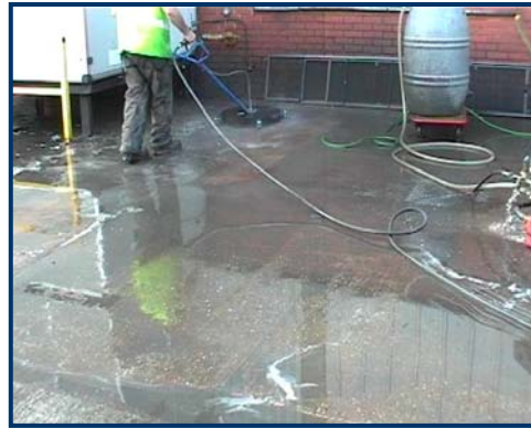
Cleaning by pressure washer
